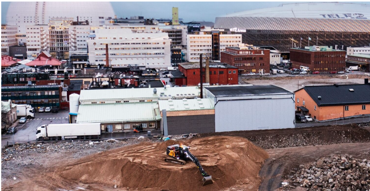
The Volvo EC230 Electric at work at Slakthusområdet
